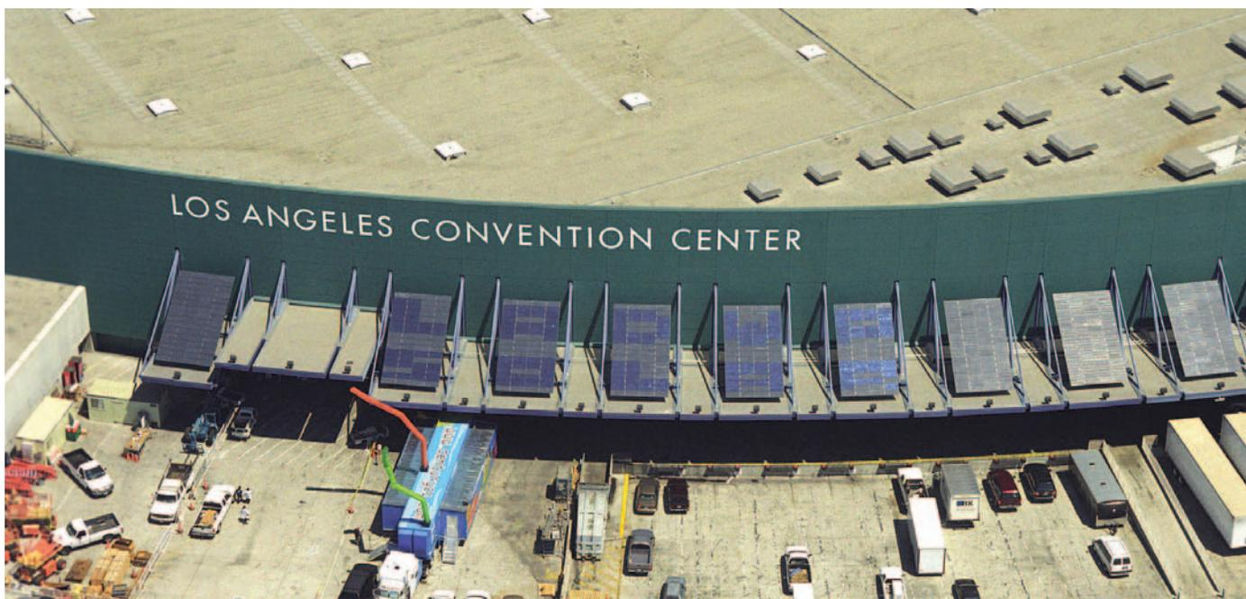
Opposite, the Los Angeles Department of Water and Power’s Temple-Duco fitness center features a photovoltaic skylight canopy. Above, LADWP has constructed a 400-kW solar photovoltaic system at the Los Angeles Convention Center.
